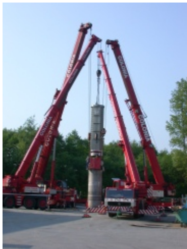
Messrs BASF Material= 1.4571 \text{\O} = 1.720 \times 45 / L = 9.238 / \text{kg} = 46.500
